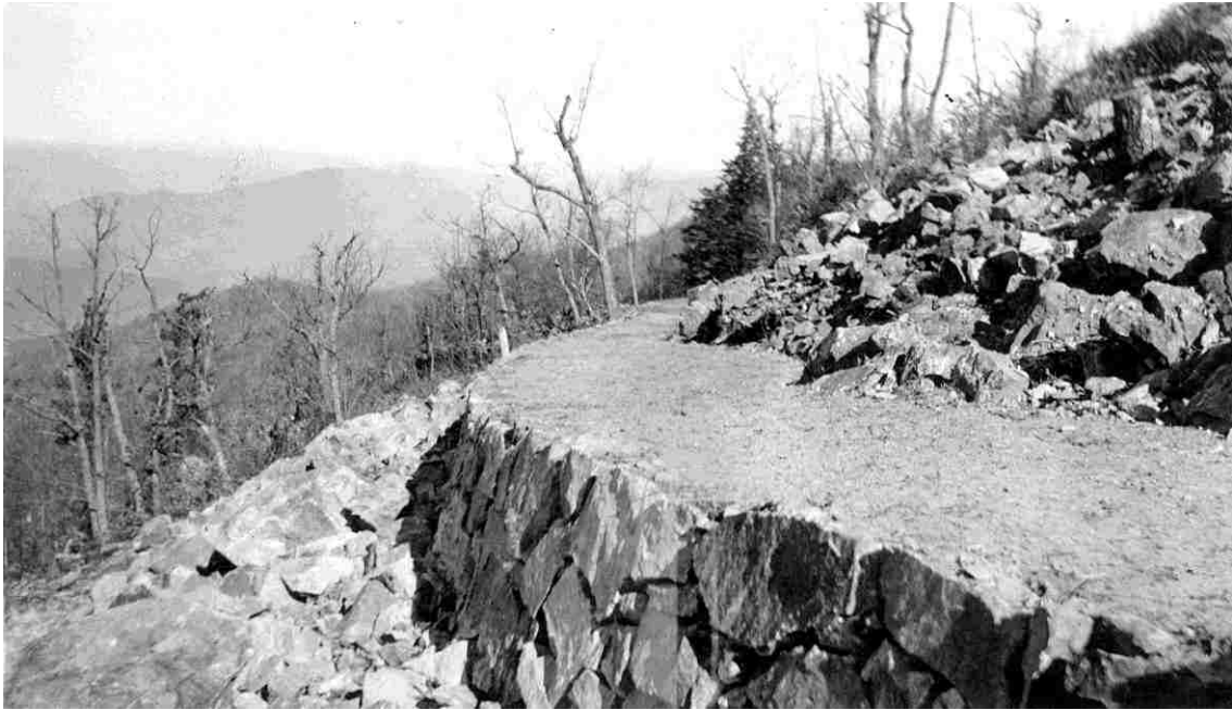
Figure 32. Graded CCC Trail, c.1936. A portion of Shenandoah National Park's relocated Appalachian Trail shows the smooth surface but unnatural appearance of graded path favored by the Civilian Conservation Corp. National Park Service.
